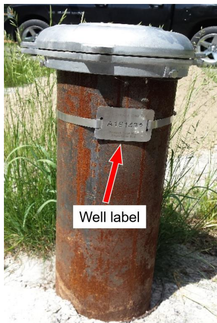
Figure 2 - Drilled well in Ontario, Canada, with well tag showing unique code (Well ID) affixed to the casing.
